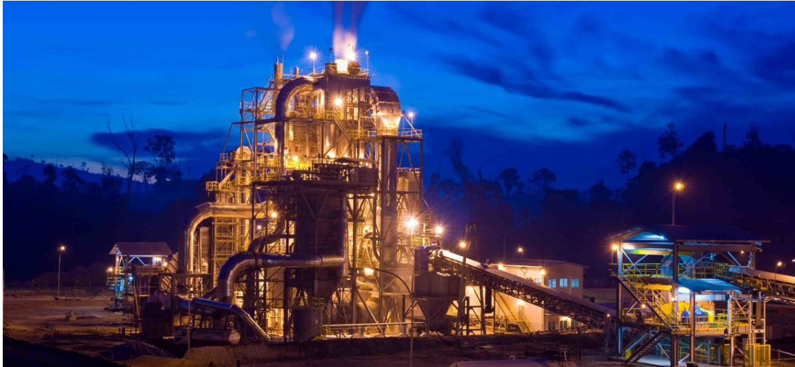
Plate 4.2. Briquetting plant at Tabang. Image taken from: https://www.thiess.com/projects/tabang-coal-processing-project/detail
