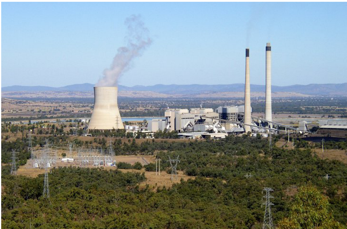
Plate 2.1. Callide power station, Queensland. Image taken from: http://www.travelling-australia.info/MainGraphics2004/P045050068Bz-750.jpg
