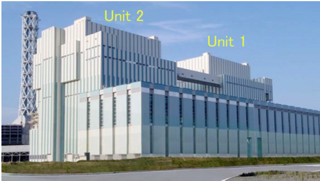
Plate 2.3 Hitachinaka Thermal Power Station, Japan. Image taken from [53].
