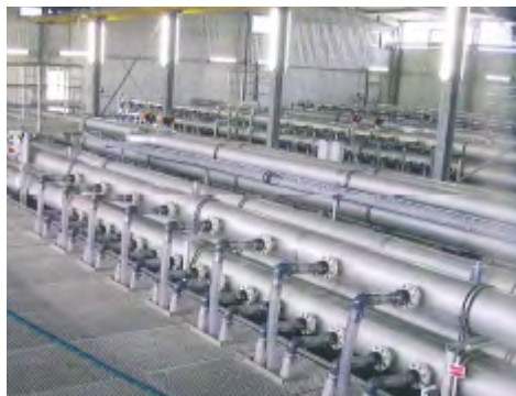
Figure 8.5 membrane installation at the WWTP Nordkanal
