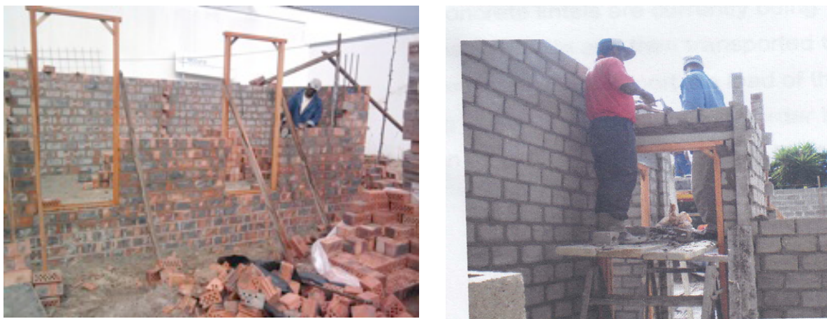
Figure 50: Brickwall and Lintel Construction
