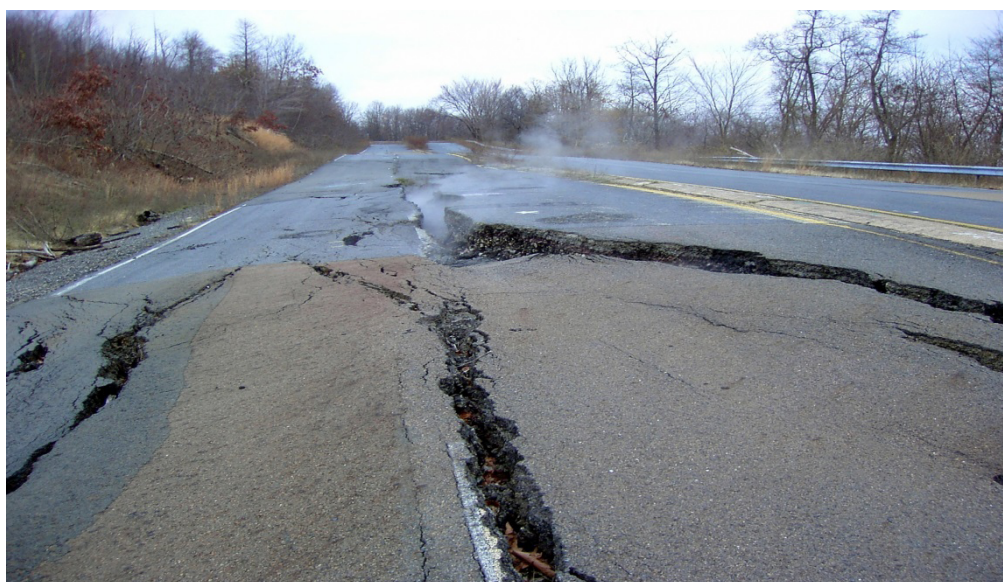
Plate 12.2. Damage to a road surface near Centralia PA due to the anthracite fire.
