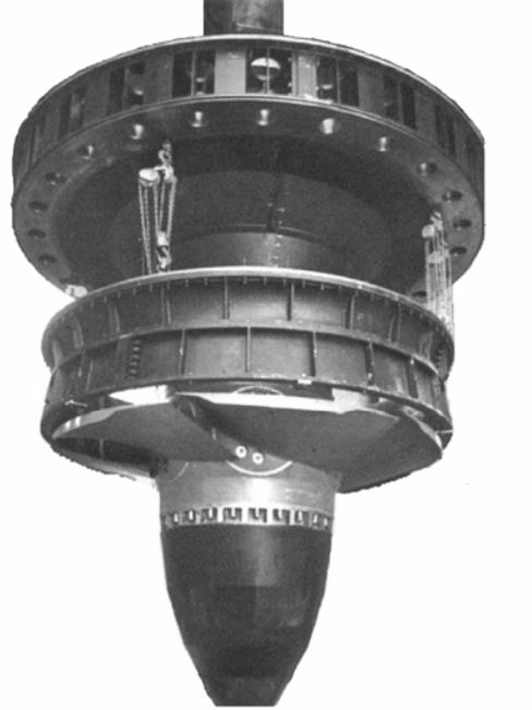
**Fig. 5.29 Fitting of the turbine rotor with cover and half discharge ring (weight 570 t)**
