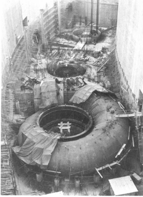
**Fig. 5.28 Sit assembly of the spiral casing (inlet diameter 10000mm)**
