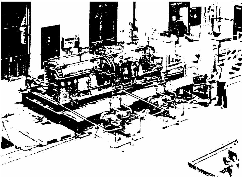
**Fig. 7.14** Two vertically split centrifugal compressors on performance test (courtesy Dresser Industries, Clark Division)
