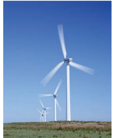
A wind farm converting the kinetic energy of the air to electrical energy. (Image Slate.)
