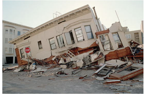
The damage to buildings constructed on water-logged loose gravel, sand, dirt and clay is greater than the damage to those constructed on hard rock. (Roger Ressmeyer/CORBIS.)
