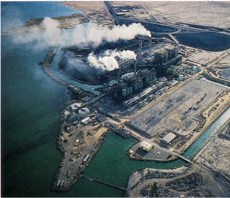
Coal-fueled electric generating plant at Four Corners, New Mexico. (Michael Collier/Stock, Boston.)
