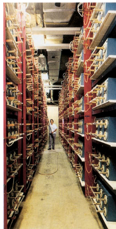
A capacitor bank for storing energy to be used by the pulsed Nova laser at Lawrence Livermore Laboratories. The laser is used in fusion studies. (Lawrence Livermore National Laboratory.)
